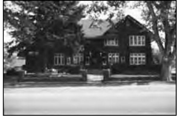
Rodman House located along Chestnut Street in Kimball, KM04-074, an example of Tudor Revival recommended as potentially eligible for the National Register
