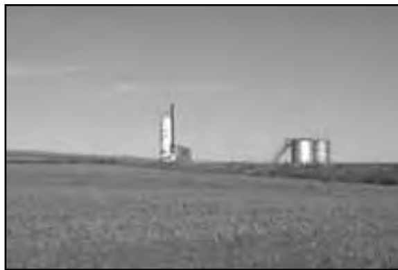
Oil storage and heating tanks, KM00-060, in Kimball County
