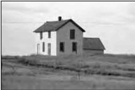
Abandoned farmstead house in rural Kimball County, KM00-012
