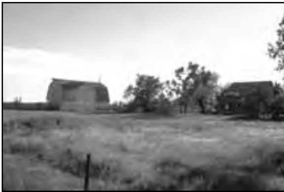
Gambrel roof barn located on farmstead near Bushnell, KM00-066
