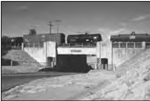
Highway 71 Underpass in Kimball, KM04-107
