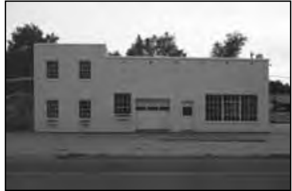
Service station located along Highway 30, KM04-159
